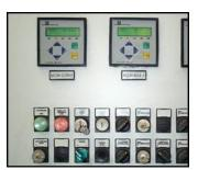
connections are made to sensors, power supply, and communication devices. A relay output is also available to control visual or audible alarm equipment, or to provide a simple input to a plant data acquisition system. Once the Artesis MCM unit is switched on, it requires minimal user configuration before entering an automated 'learn' mode during which the complete normal operating condition of the connected system is established. This process accommodates the full range
